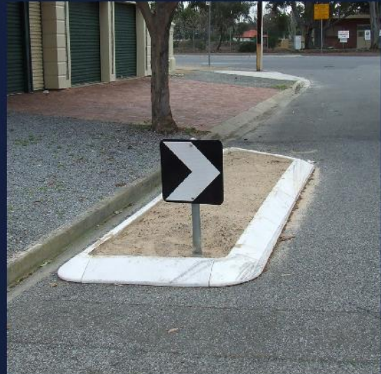
Installation of Traffic Calming Kerb Blisters
